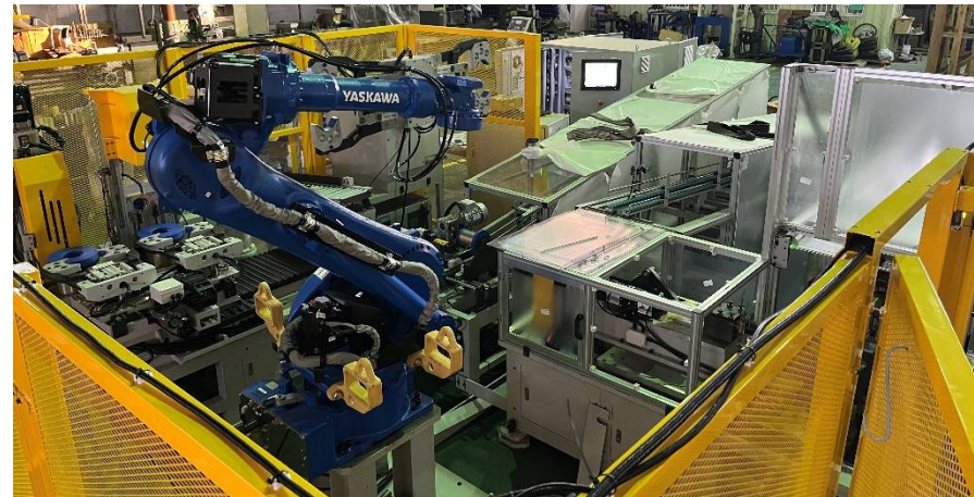
GBD Canning Line -Shell Seam Tracking/CCD Check -Monolith and Mat Measuring ST -CCD Check/Monolith and Mat Wrapping -Shell and Wrapped Monolith Stuffing -GBD Calibration (Shrinking) -GBD Check/Laser Marking/QR Code Reading -Handling Robot for Automation
